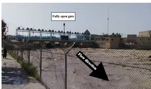
Fig. 6 View downstream of Zahak Dam during the flood of the 2018-2019 water year
