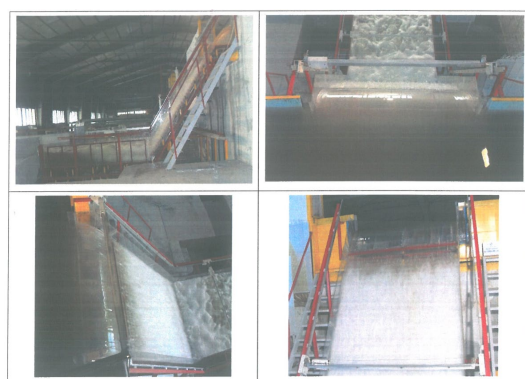
Fig. 6 Flow pattern on the spillway sill, stepped rapids and the stilling basin
